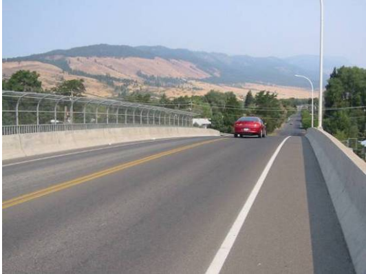
Facilities such as roadway shoulders accommodate bicycle travel and provide a safe location for disabled vehicles to stop
